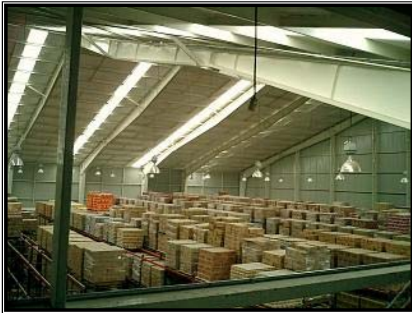
Interior de la nave principal
