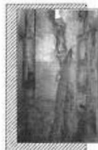
SE PRESENTA UNA CRACK, CON UN DESPLAZAMIENTO MÁXIMO DE 1.00M, LA MADERA DE LA VENTANA ESTÁ EN MALAS CONDICIONES.
