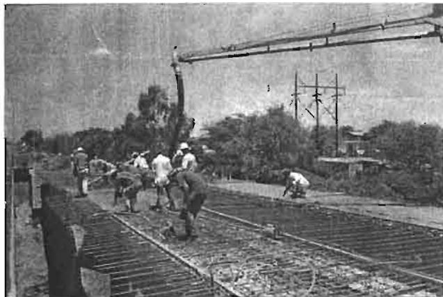
COLADO DE LA LOSA TAPA DE TRABES CON CONCRETO  $f'c=300$  kg/cm<sup>2</sup>.
