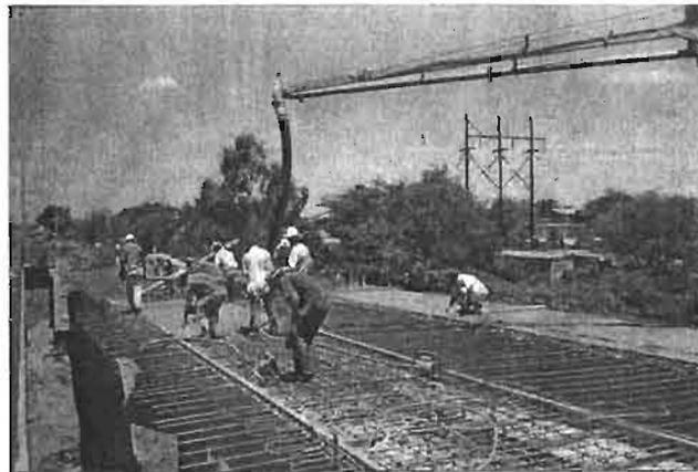
COLADO DE LA LOSA TAPA DE TRABES CON CONCRETO  $F'c = 300 \text{ kg/cm}^2$ .
