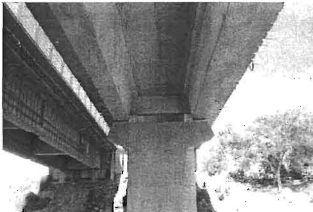
DETALLE DE LOSA CENTRAL DONDE SE APRECIA EL DIAFRAGMA TERMINADO.
