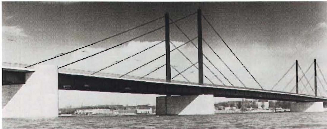
Fig. 1-32 North Bridge , Dusseldorf, Alemania [Ref. B-25].
