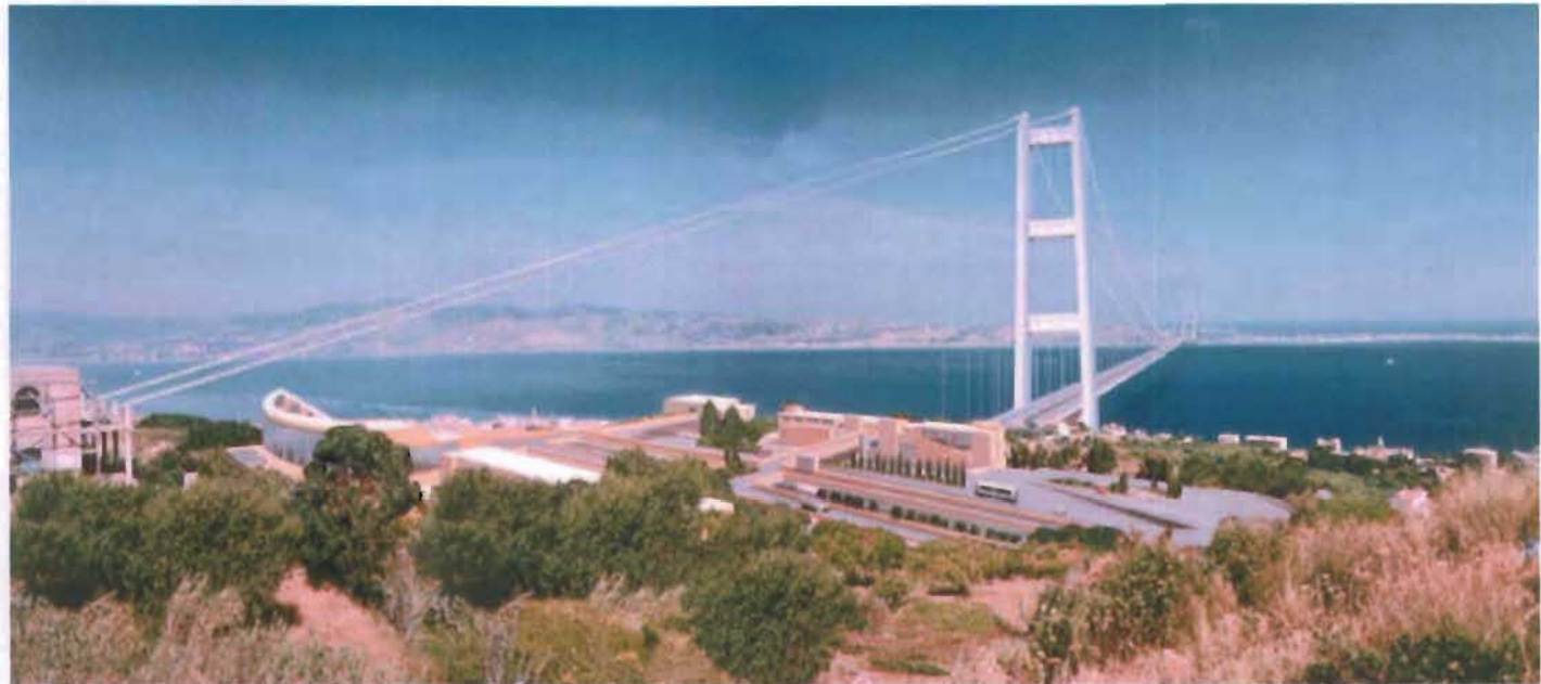
Fig. 1-46 Puente Messina 38 , Italia [Ref. B-6].
