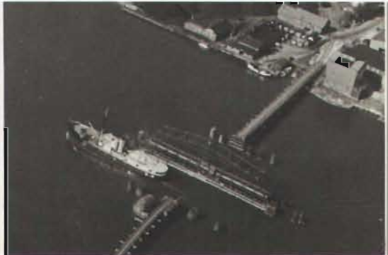
Fig. 1-12 Sturgeon Bay, Swing Bridge [Ref. B-29].
