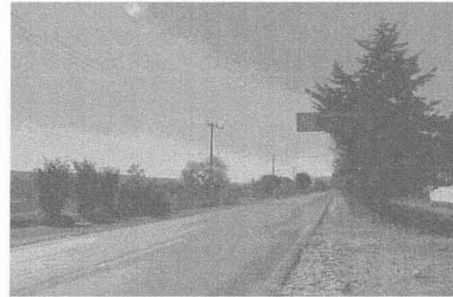
Carretera Federal No. 115 México-Cuautla
