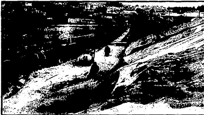
FIGURA 5.23 "COMPACTADO DE ARENA TÉRMICA CON RODILLO LISO
