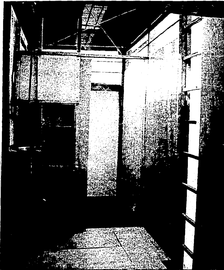
VISTA PRINCIPAL INTERIOR
