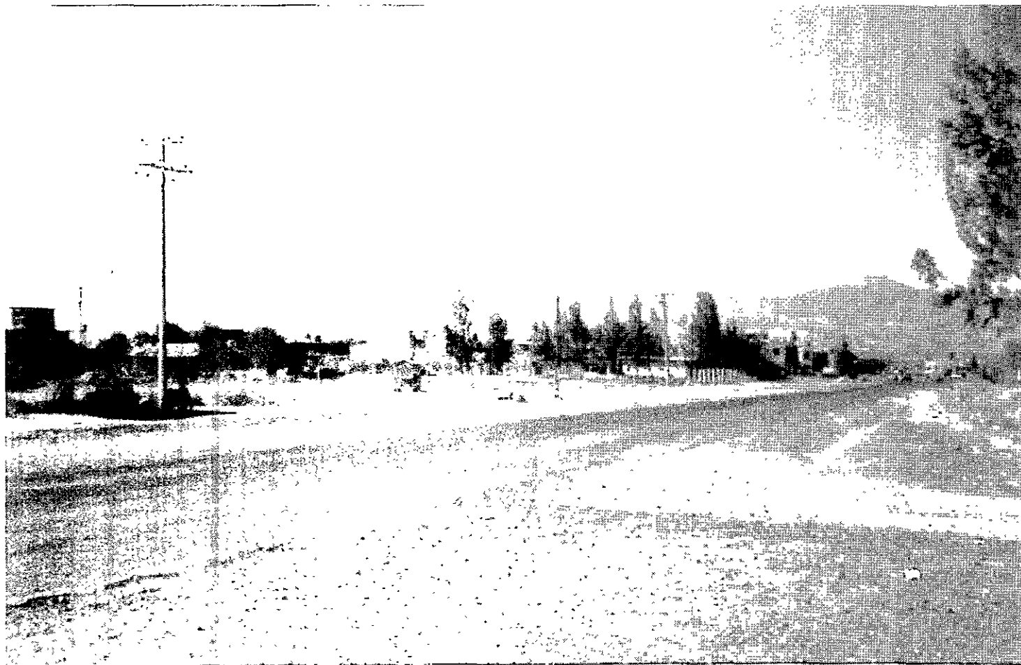
CARRETERA FEDERAL PATZCUARO-MORELIA.
