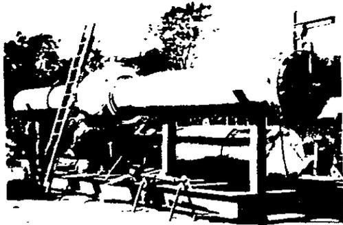
A complete skid-mounted 30" receiving module. This system was supplied with all associated piping, a 36" diameter drain sump tank and weld in ball valves for mainline piping. Barrel is a 34" OD with 300 lb quick opening closure.
