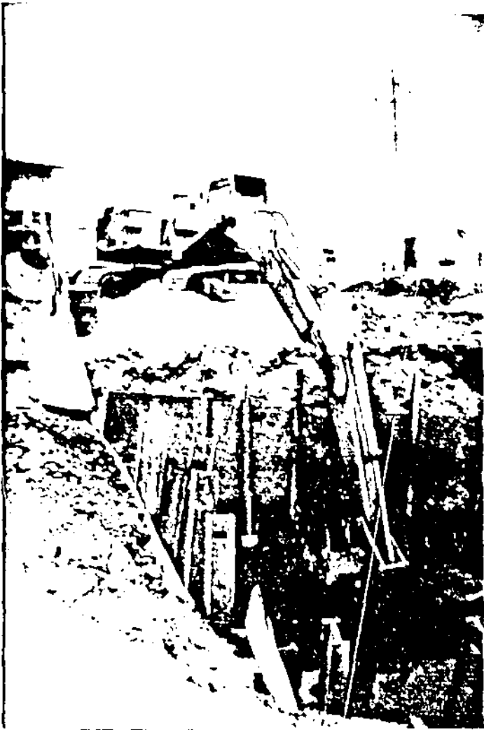
FOTO No. 21 - Excavation site showing trench and shoring.
