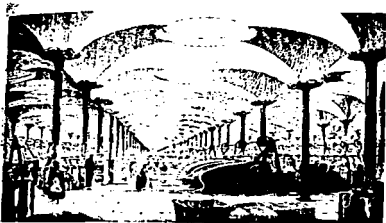
The Great Hall of Marshall's Gas mill at Leeds, c. 1870. Although a 'late' piece, the illustration well illustrates the separate pieces of belt-driven machinery with the operators at work under their overcast. From Great Industries of Great Britain , London, undated.
