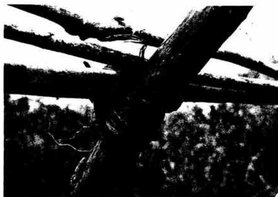
Fig. 6. Fresh leaves baked directly over fire and cut in strips to be used to tie the roof thatch of houses.
