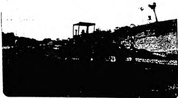
FIG. 5.1 MEZCLA EN EL LUGAR CON MOTOCONFORMADORA
