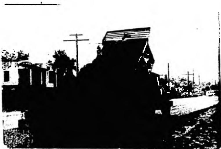
FIG. 5.3. TENDIDO DE LA MEZCLA
