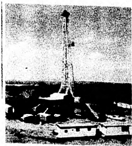
ANTENNA AT STATION
